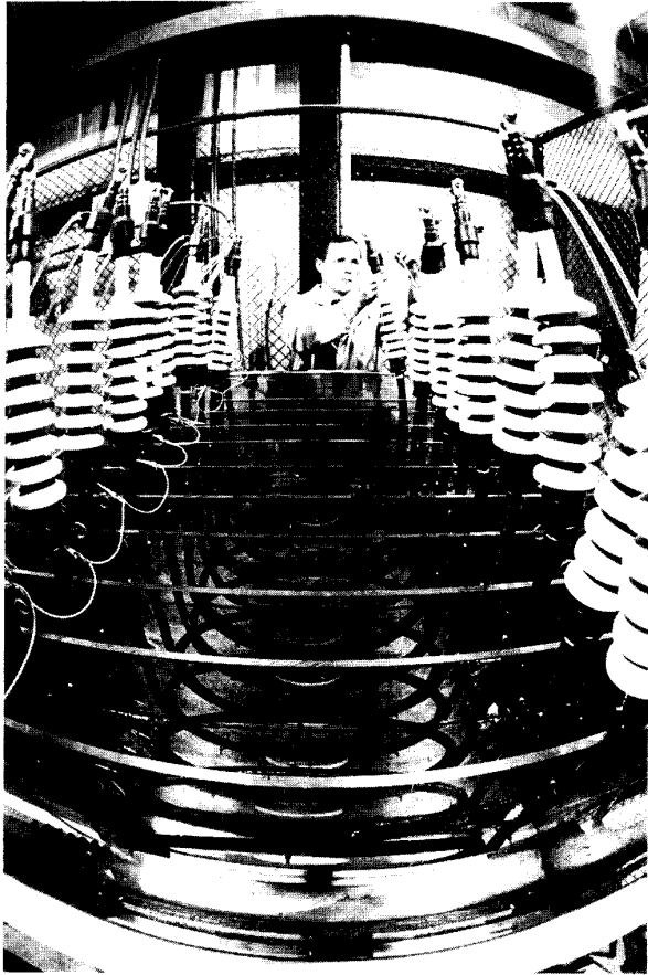
Fig. 2. The Du Pont Company is spearheading the industry's newest ACLT for URD cable. The cables, some with insulation based on Du Pont "Nordel"® hydrocarbon rubber, are energized with 35 kV and 250 A in a cycle schedule of 8 hr on and 16 hr off while immersed in a controlled, deionized water-bath. The test measures the retention of dielectric strength as the cable specimens undergo accelerated thermal, mechanical, and electrical stress conditions.
